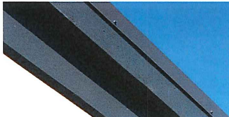
6. COMBFACED WOOD FASCIA + METAL FLASHING
