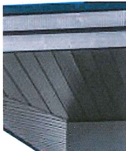
7. PERFORATED ALUMINIUM SOFFIT, CHARCOAL
